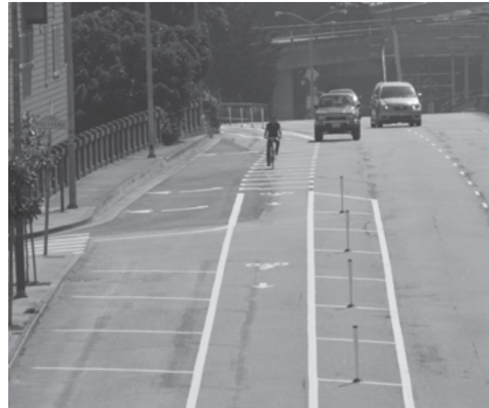
San José Avenue is soon to see concrete safety barriers added to increase the comfort and safety of biking.
