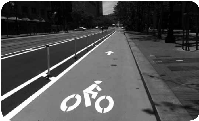
Market Street was repaved this June between 6th Street and Van Ness Avenue.
